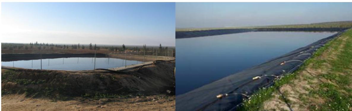
Photo 1: VW storage basins
