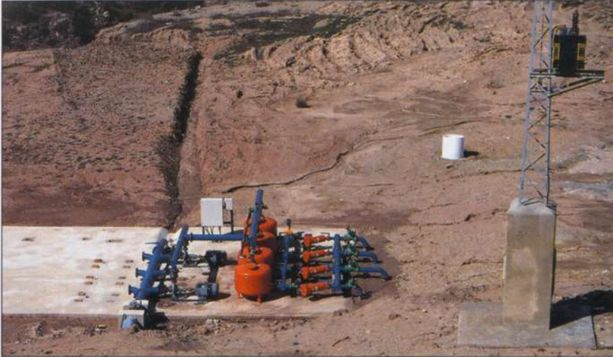
Water filtering equipment for drip irrigation. Both sand and mesh filters are used to ensure proper functioning.
