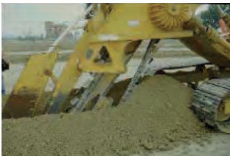
Figure 23. Digging and laying drainage pipes.
