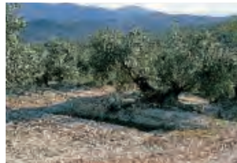
Figure 29. Olive tree with trench dug with a back digger to harvest water and sediment.
