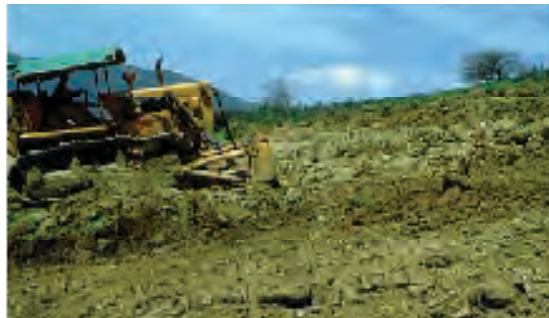
Figure 20. Levelling the site.
