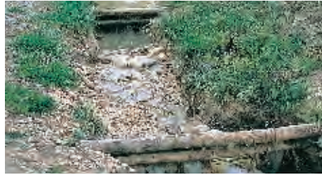
Figure 30. Small gully with spontaneous vegetation and small structures to slow down runoff velocity.
