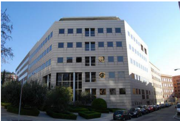
■ The International Olive Oil Council's headquarters in Calle Principe de Vergara 154 in Madrid
